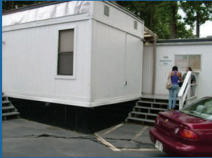
Old clinic located on the Elizabeth Inn Campus
